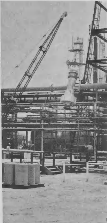
The tip is carefully inched upwards, with final adjustments made by CB&I man...
